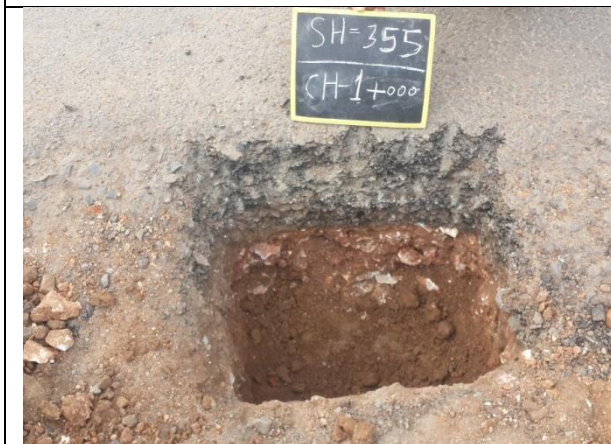
Road site Pit excavation for pavement crust measurement
