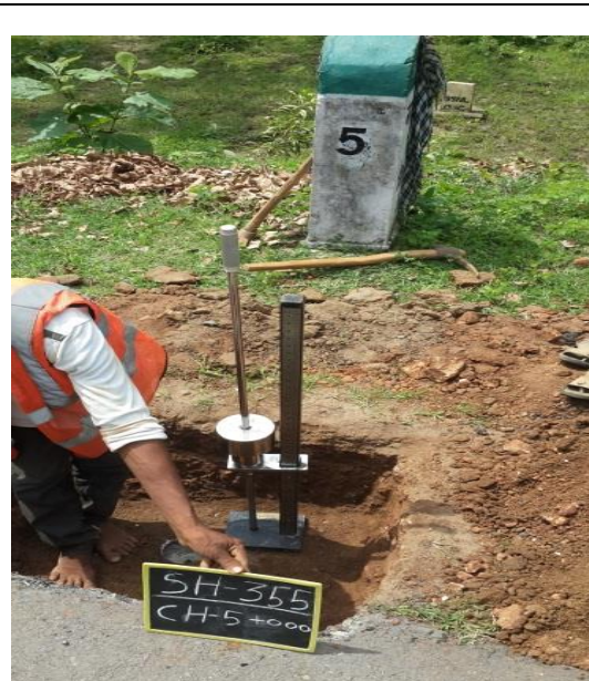
DCP Test in progress
