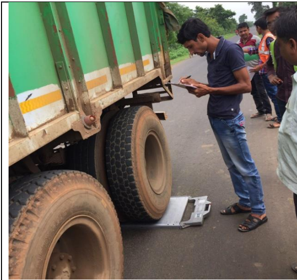
Axle Load Survey in progress
