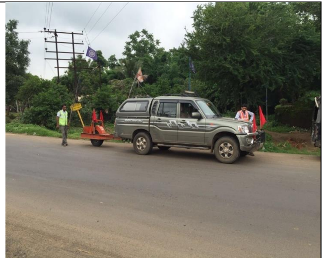
Surface evenness and roughness survey in progress
